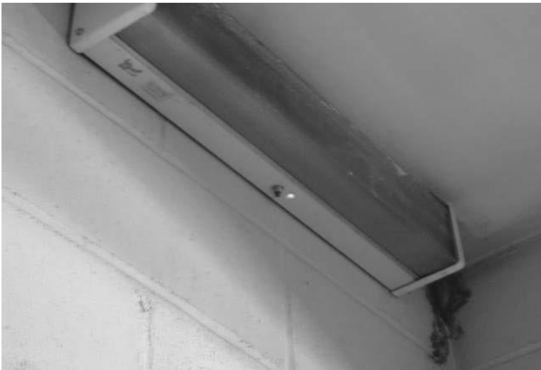
Inside:Emergency Power-Auxiliary Lighting Inoperable- Working test button but not light.
