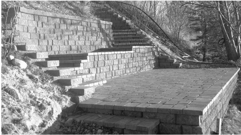
Guardrail missing or not installed (Patio)
