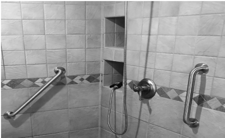
Grab Bar must serve its intended purpose and not have hazards or damage.
