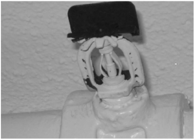
Sprinkler assembly has evidence of foreign material that is detrimental to performance
